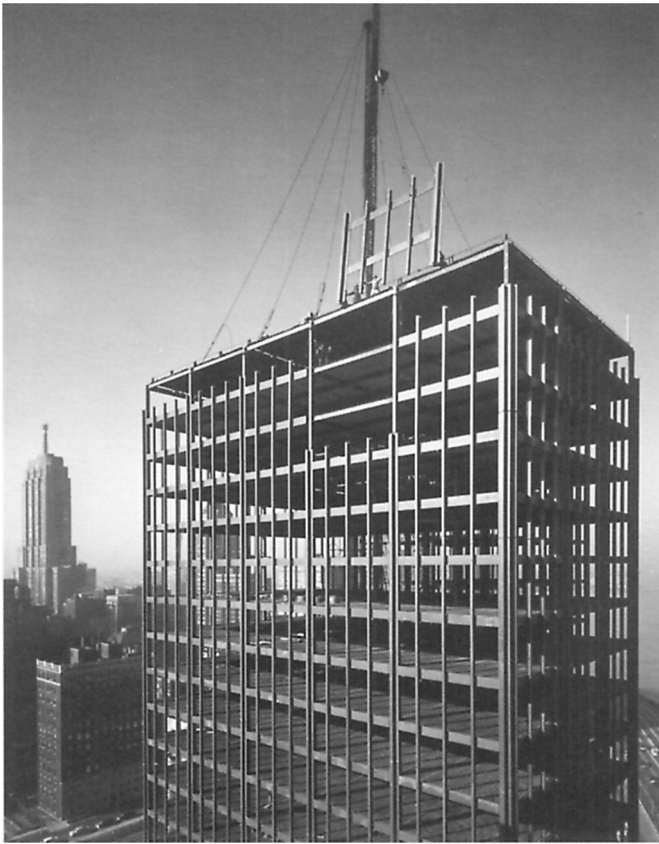
29. Mies, 860–880 North Lake Shore Drive, 1948–51, under construction
